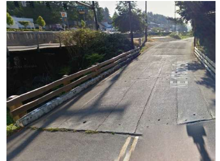
Figure A: Existing Bridge
