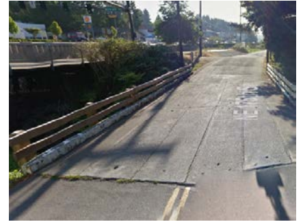
Figure A: Existing Bridge
