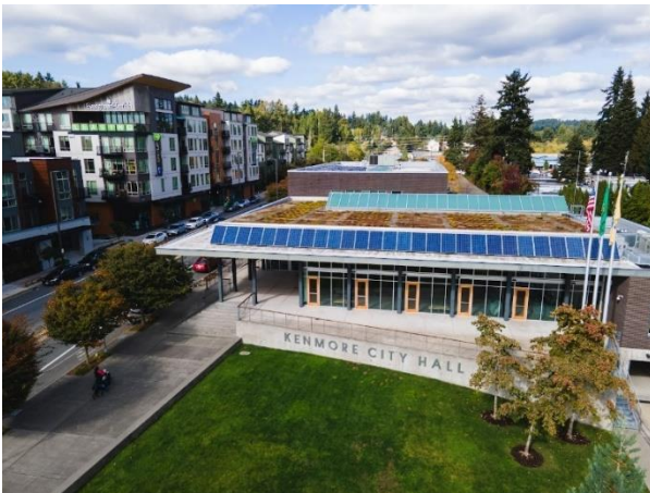
Existing solar on City Hall
