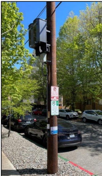
Examples of pole charger installations
